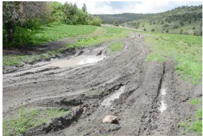
The damage at this site has recently gotten worse, because the emergency closure enacted three years ago is no longer being implemented.
